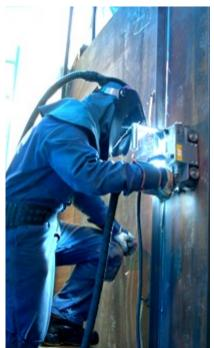
Vertical up butt welding using guide rail
